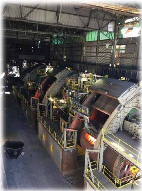
HAYDEN SMELTER – NEW CONVERTER AISLE
