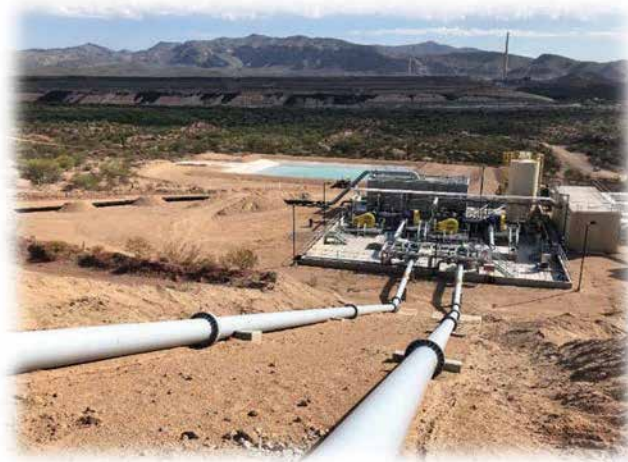
NEW TAILINGS PUMP STATION FOR CONCENTRATOR
