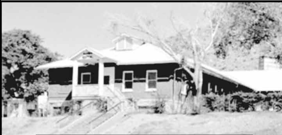
Magma Hospital, Superior, Arizona
