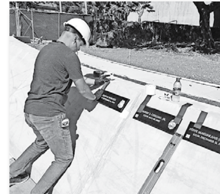
Working on the Fallen Officer Memorial.
