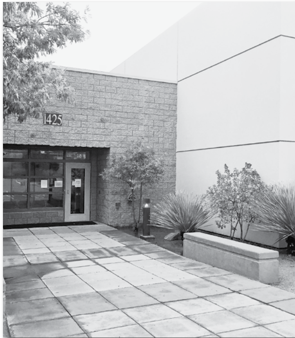
Gila County Juvenile Detention Center is no longer open.
