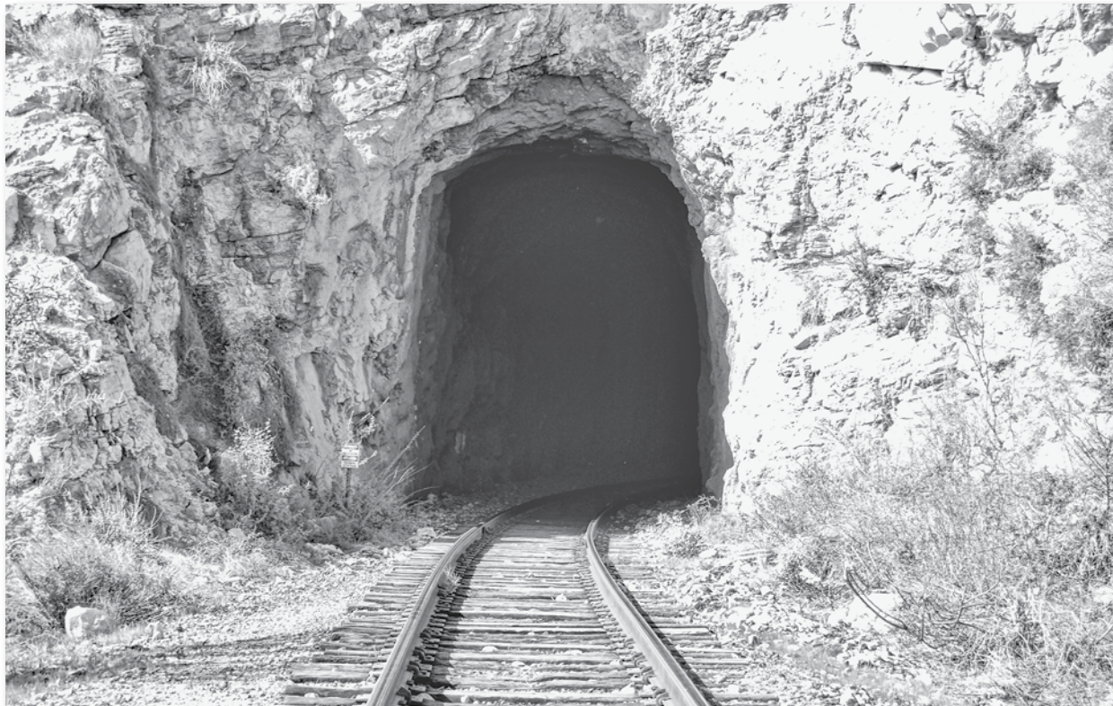
A tunnel on the Copper Basin Railway, still in use today.
