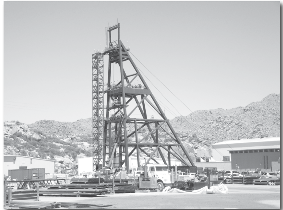
The headframe at Resolution Copper's primary shaft near Superior.
