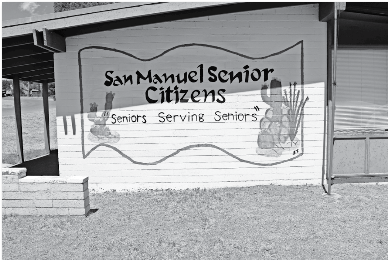
The outside of the San Manuel Senior Center will also receive some much needed attention with the creation of a parking lot and making the outside ADA compliant.
