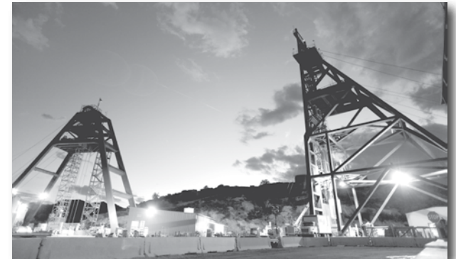
A view of headframes at Resolution Copper.
