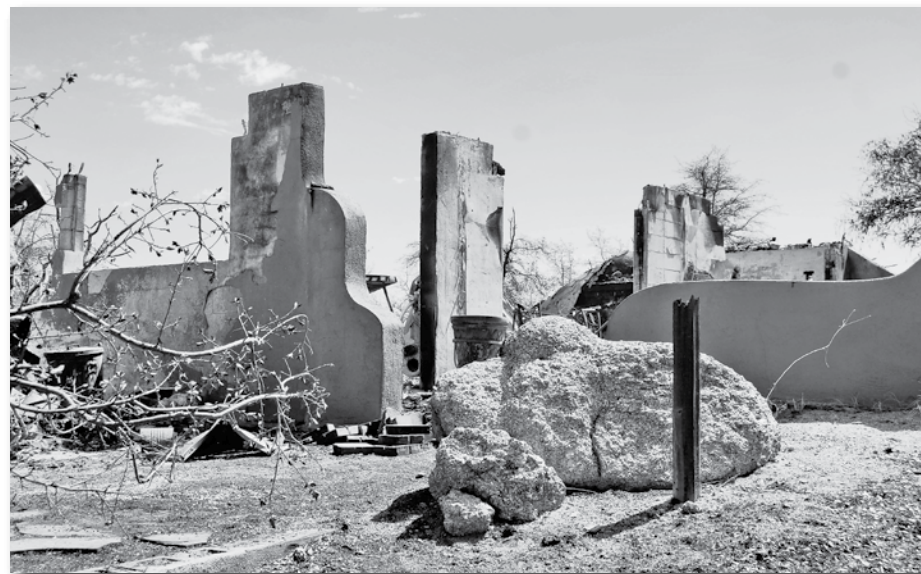
Only a few walls remain after a wildfire destroyed the Chatham residence.
