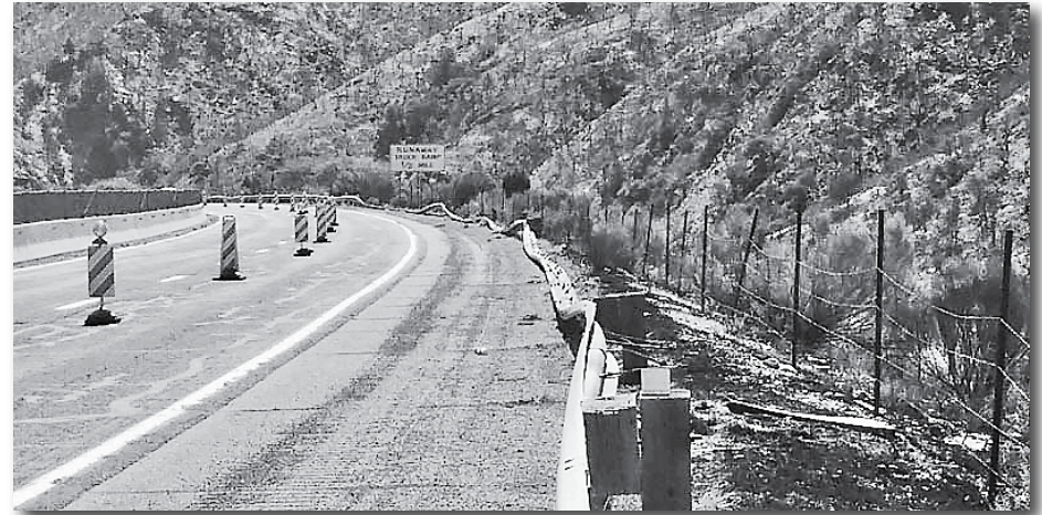
Guardrails on SR 87 south of Payson damaged by wildfire in 2020.
