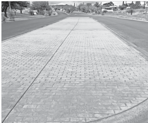
Stamped concrete median at the entrance to San Manuel.
