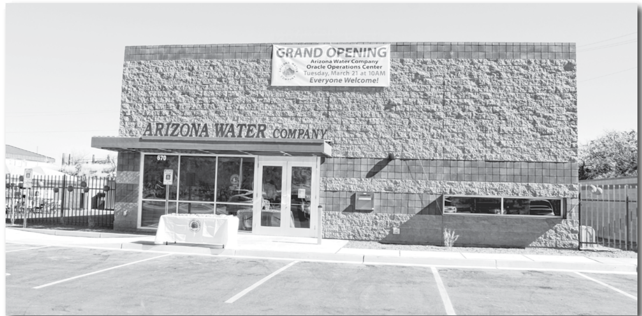
Arizona Water Company’s new Oracle Operations Center celebrated its grand opening last week. The company said the new facility will save them money in the future.
