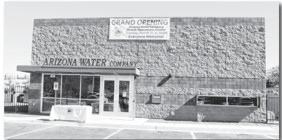
Arizona Water Company's new Oracle Operations Center had its grand opening last week. The company has said that the new facility will help trim operating costs in the future.
