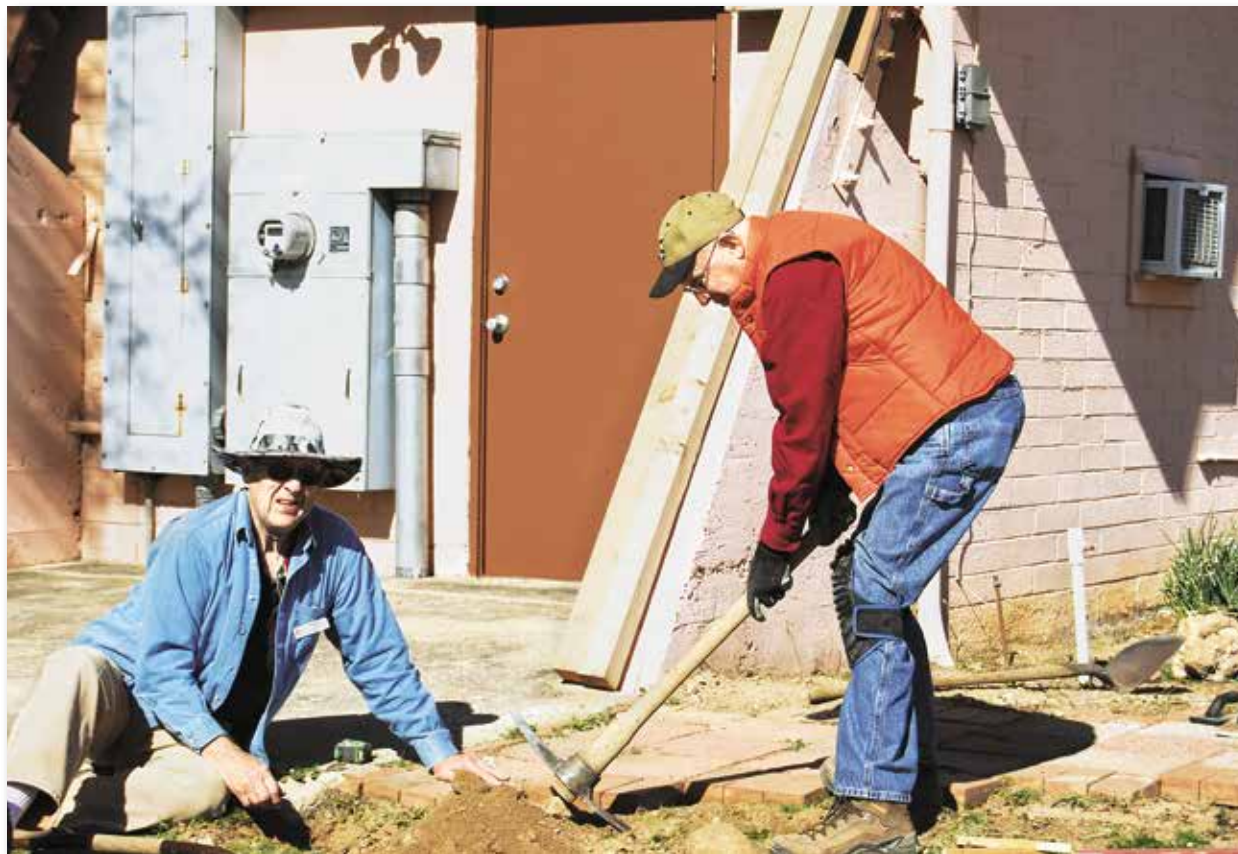
Bob Bontz and Paul Hope restoring gutter system.
