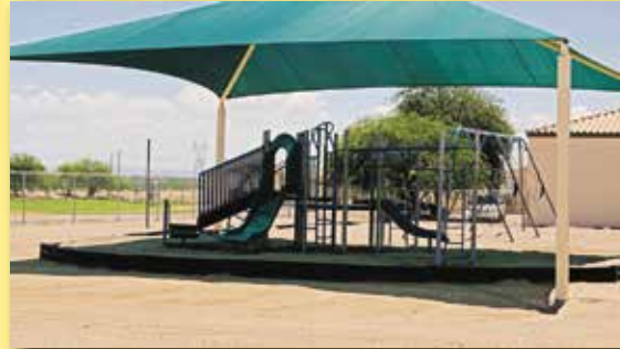
Another shaded playground area on the S.T.E.A.M. Prep Academy campus.
