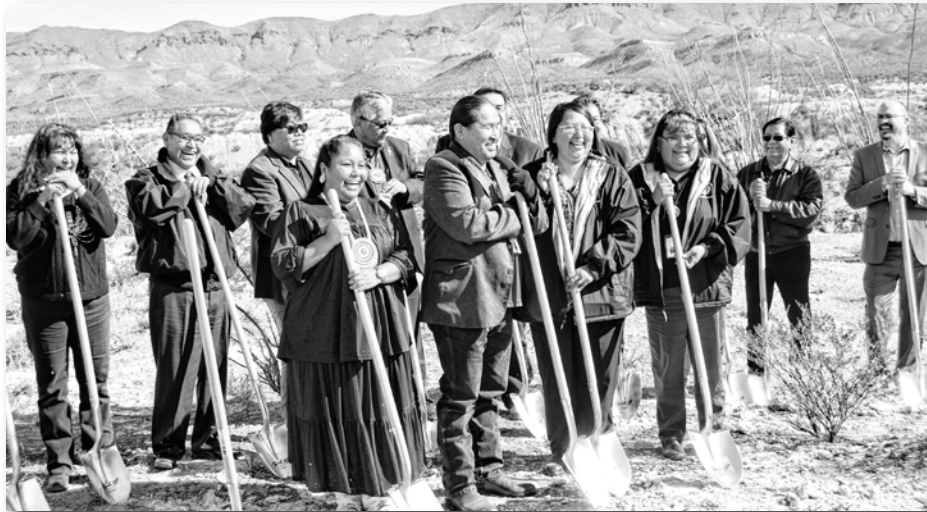
Leaders from the San Carlos Apache Tribe as well as local leaders officially broke ground last week on the Apache Sky Casino near Dudleyville. They plan to open in June. John Hernandez | CBN
