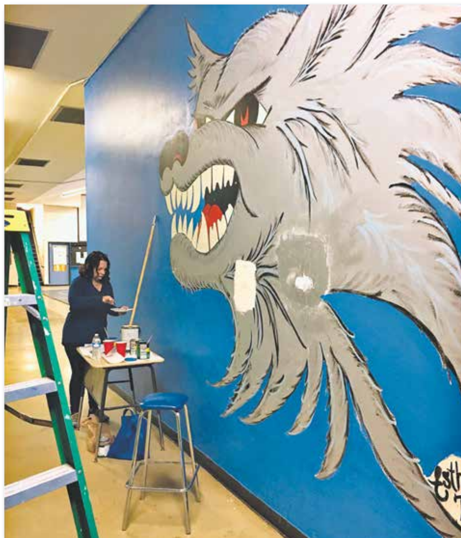
Jennifer Suarez repairs her mother's mural at Hayden High School. Esther Yanez is the original artist.
