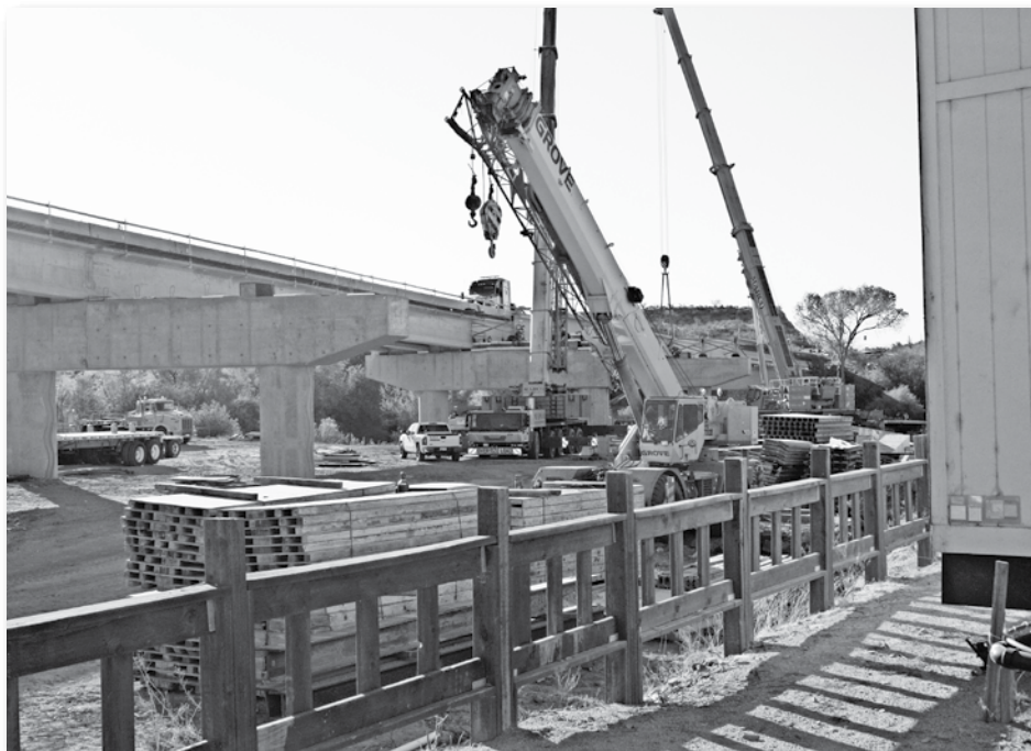
Construction workers carefully place bridge girders on the new Winkelman Bridge on SR 77.
