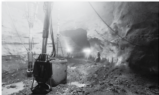
The last blast zone at the bottom of the shaft.
