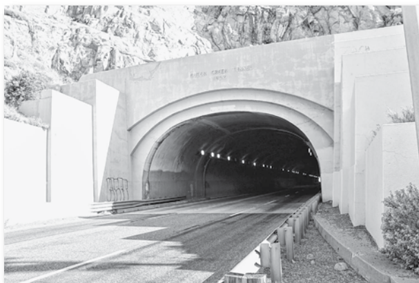
US 60 Queen Creek Tunnel.
