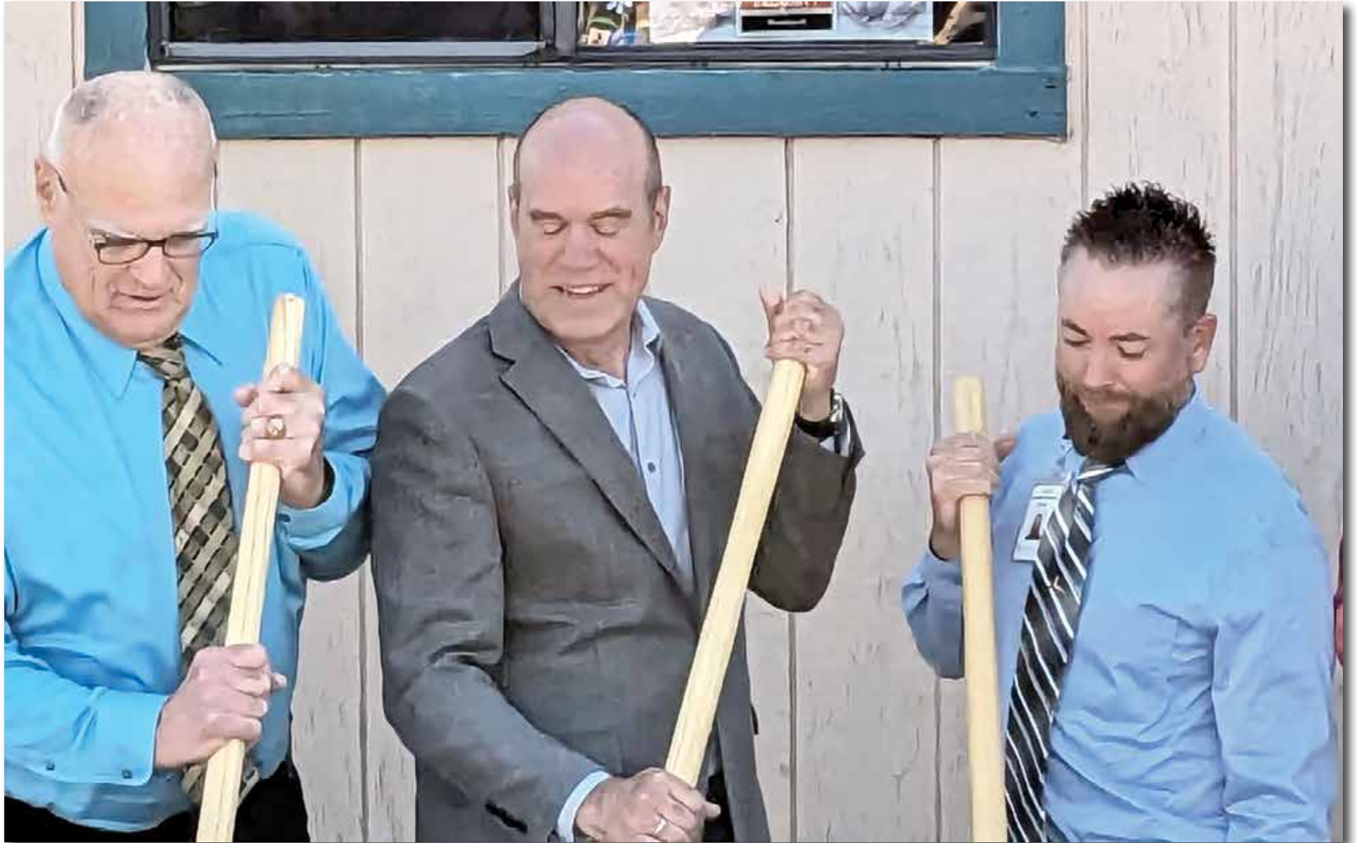
Dave Orzell (left) of the Copper Basin Health Foundation, Neil Terry with Orcutt Winslow Architects (center) and Tanner Carlson, PA, of Cobre Valley Regional Medical Center are ready to break ground for the new Kearny Clinic.
