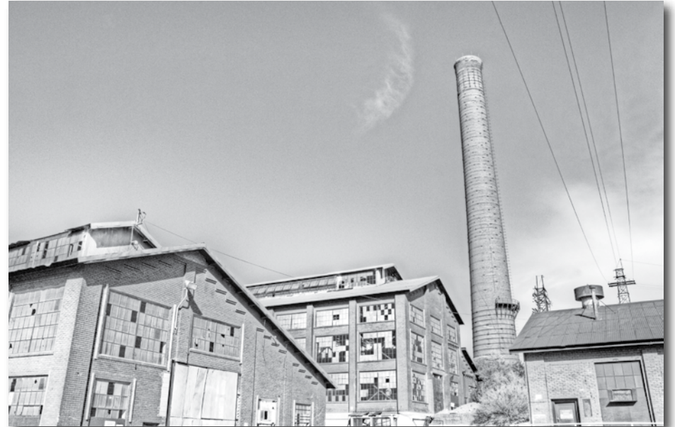
The Historic Magma Copper Smelter Complex in Superior. The stack is set to be demolished this weekend. Cat Brown | Copper Area News
