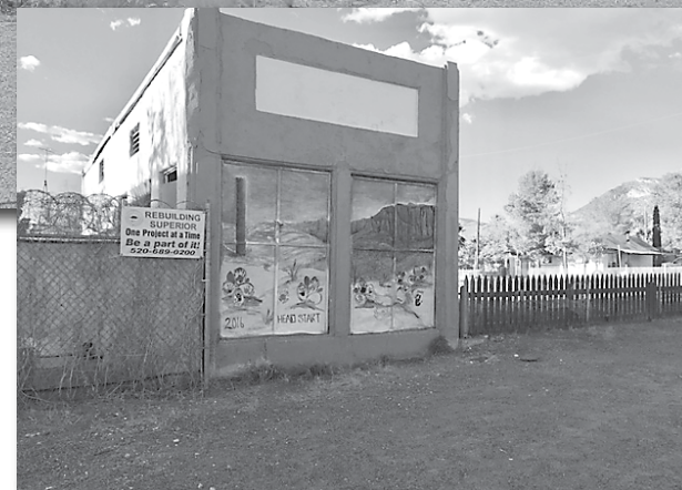
Payer Motors before (above) and after (right) a mural was painted onto the boarded up windows.
