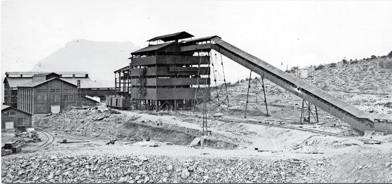
Roaster at Magma smelter during construction c. Dec. 1923.
