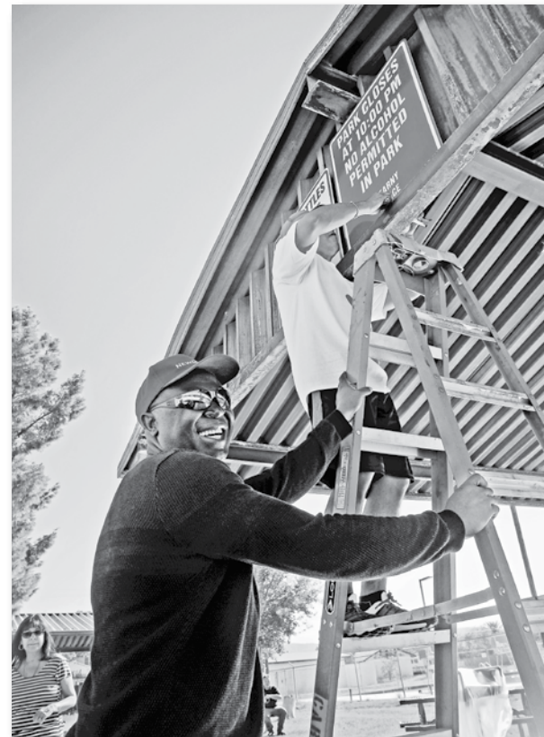
Preparing the Ramada for paint.
