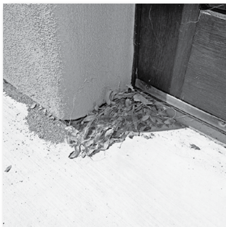
Once ignited by embers, little brushy pockets like this can lead to a greater home fire. Holt Bodinson | Submitted
