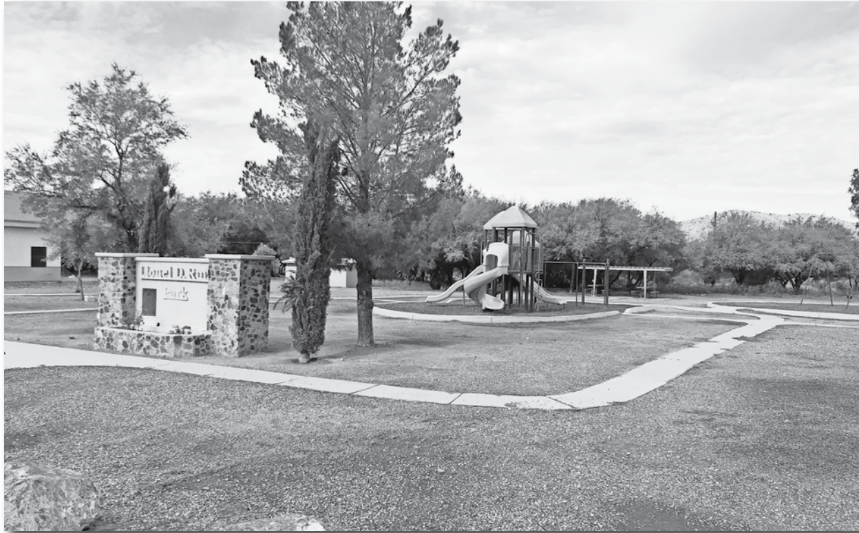
The Lionel D. Ruiz Park in Dudleyville will be receiving some upgrades for ADA compliance.
